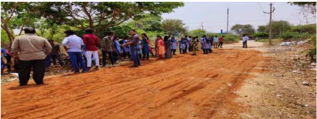
Students and Staff at repairing the ROAD
