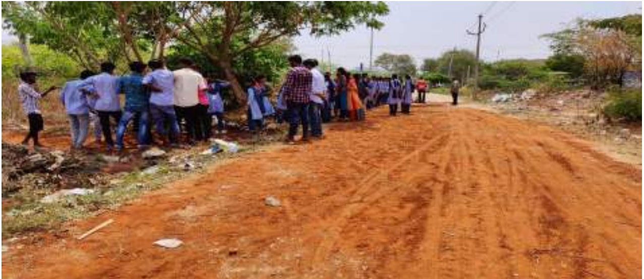
After Repair the Road
