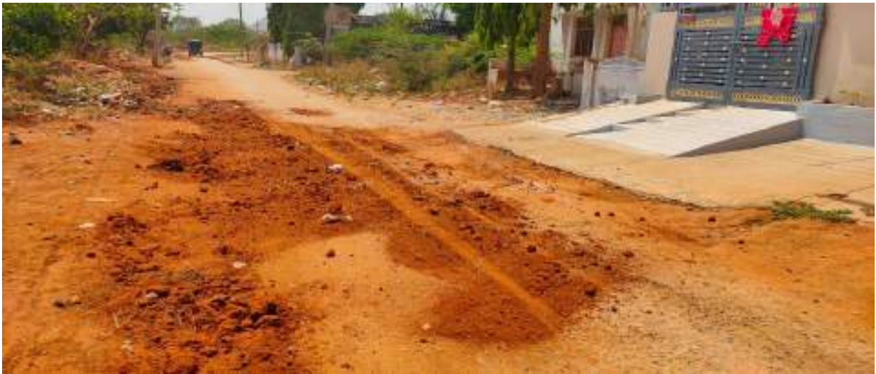
Filled with Gravel and Sand on the Road Pits
